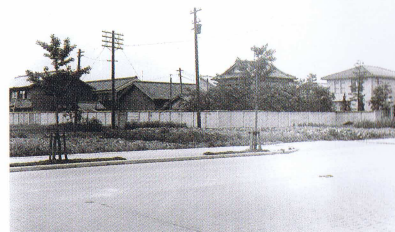
1930(昭和5)年頃の社屋 Kashifuji factory during the 1930s
